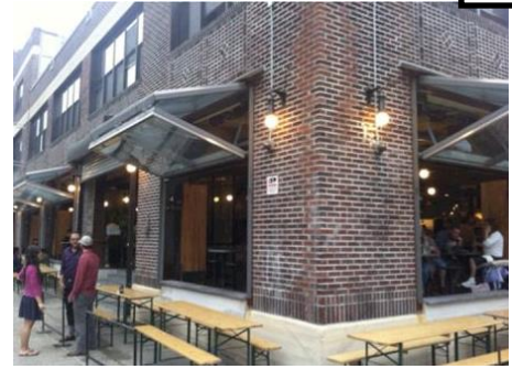
Example: Operable Windows and Overhead Doors
